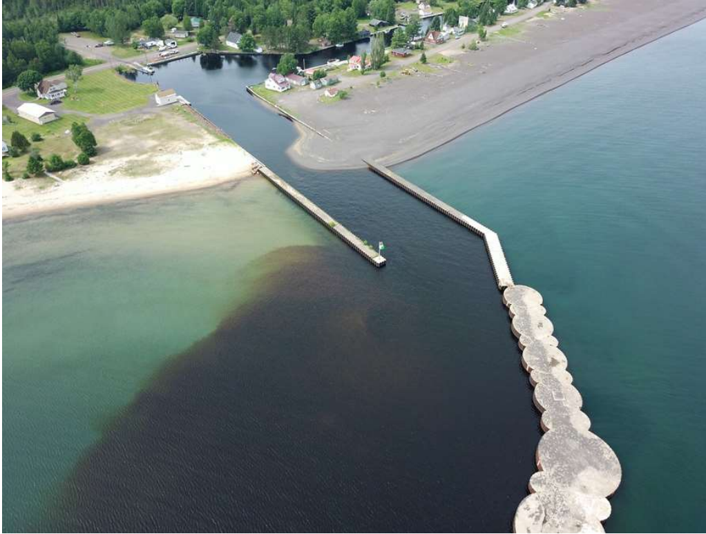
Figure 2.4. Image drone shot of Traverse River seawall
