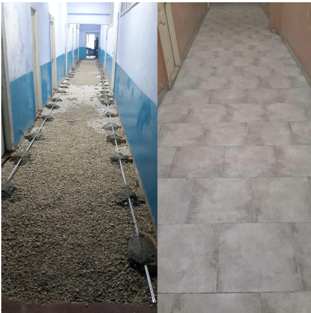
Figure 5: The image shows the access hallways after the rotten floors were removed. The floor was leveled and filled in with gravel and then concrete was poured over. Durable tiles were added along with a new coat of paint.
