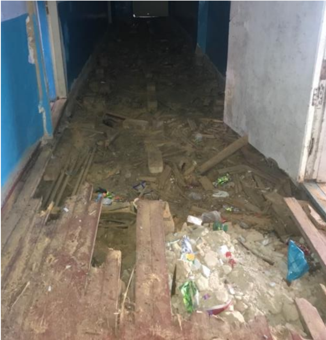
Figure 3: The image shows the condition of the access hallway to the gym. As shown in the image, the floor is rotten and in most areas missing.
