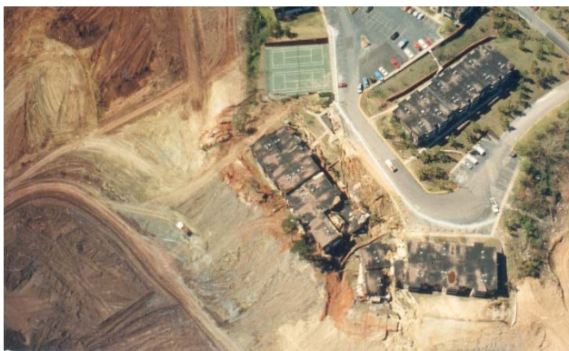
FIGURE 1: THE MOUNTAIN TOP APARTMENTS AND THE CONSTRUCTION SITE DIRECTLY AFTER THE TWO GROUND MOVEMENTS.
