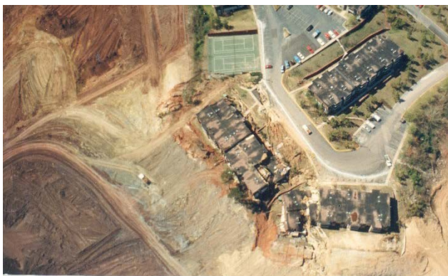
FIGURE 1: THE MOUNTAIN TOP APARTMENTS AND THE CONSTRUCTION SITE DIRECTLY AFTER THE TWO GROUND MOVEMENTS.
