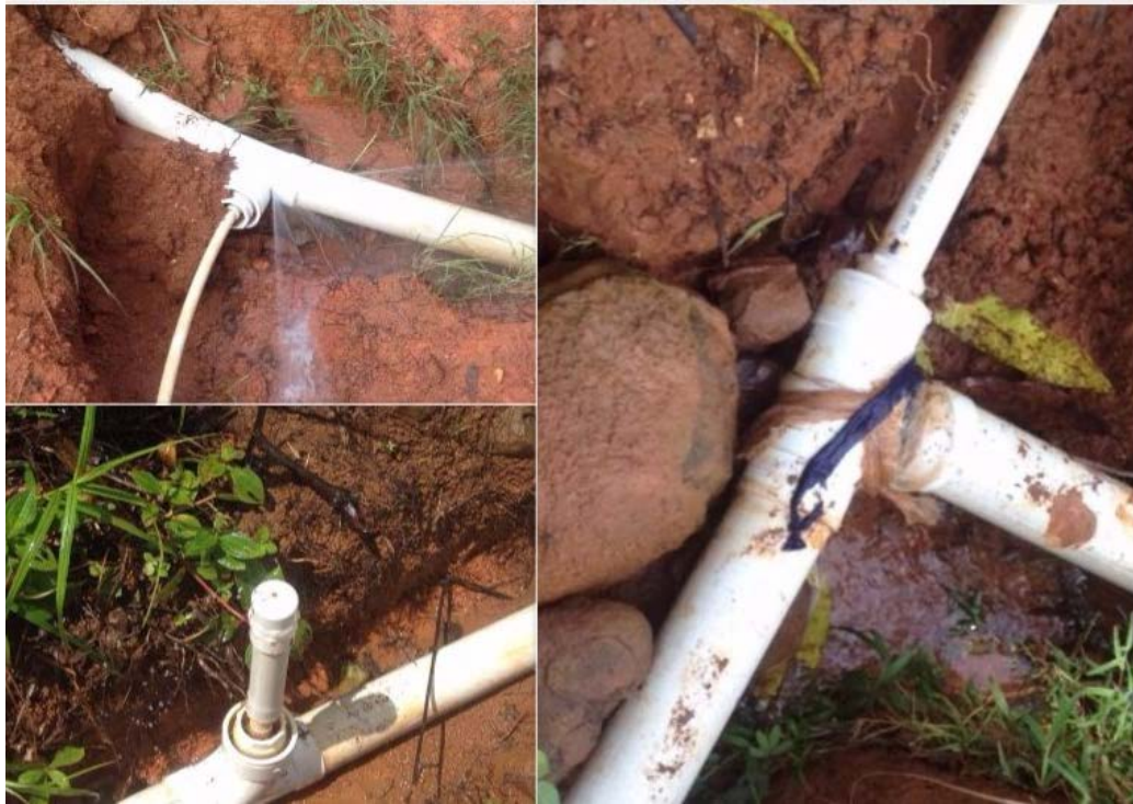
Figure 4.1. Leaks Observed during Inspection of the Espavé Water System on November 6, 2015. Clockwise from Top Left: Reduction Leading to P10 spraying water; Leak at Junction N9 Wrapped in Plastic; Air Release valve under high pressure spraying water. (Photos by author)
