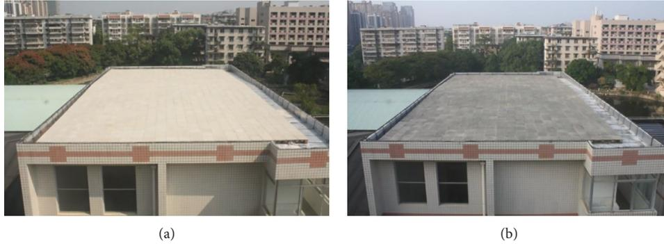
FIGURE 1: Concrete tiles are widely used as the overlay of a flat double-skin roof in Southern China. (a) A new concrete tile roof. (b) 2-3 years tile roof: the tiles have been darkened by dust deposit and algae growth.
