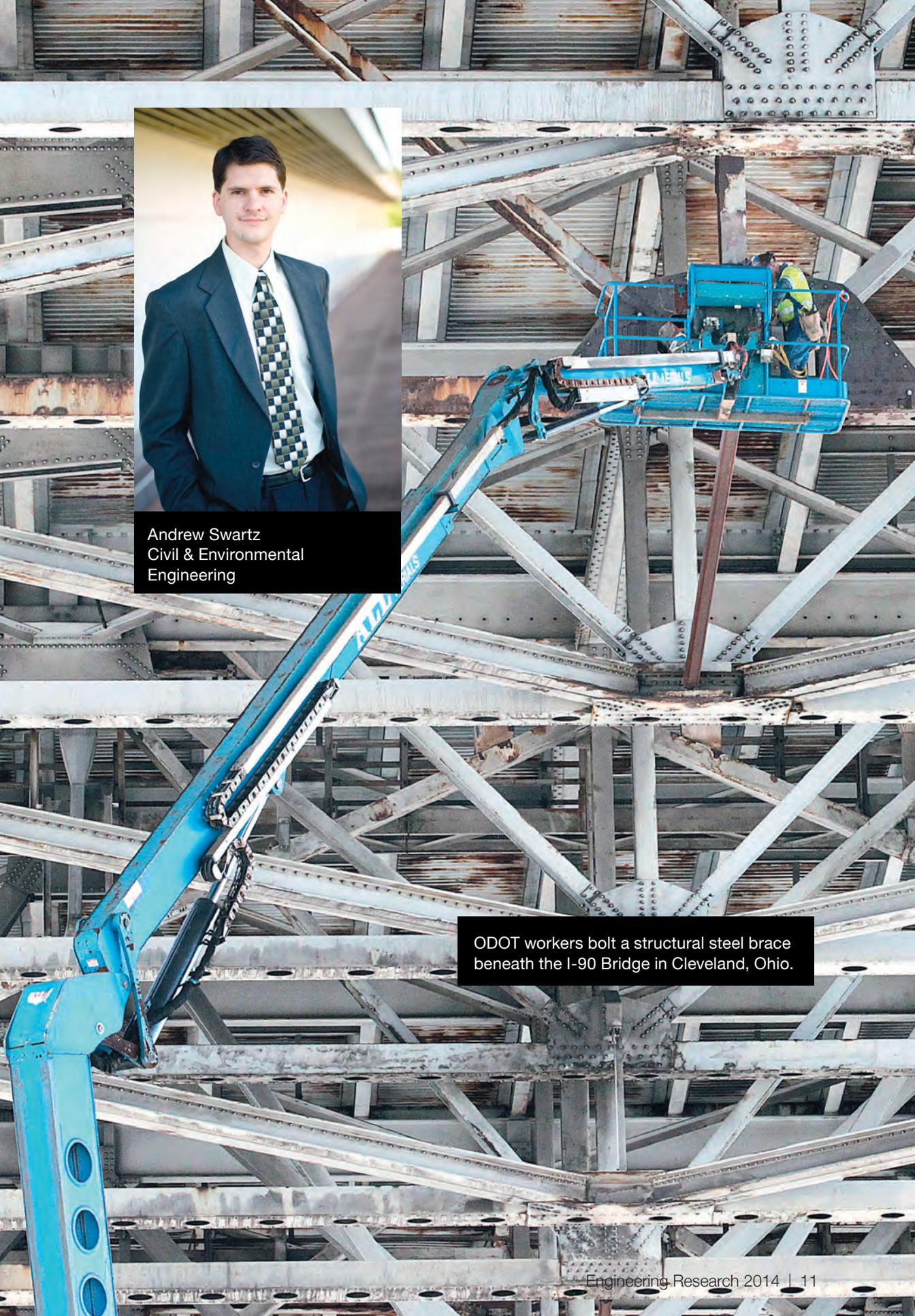
ODOT workers bolt a structural steel brace beneath the I-90 Bridge in Cleveland, Ohio.
