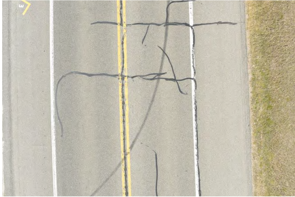
Figure 20: Nikon D810 image of Holton Rd collected via UAV showing sealed crack details.
