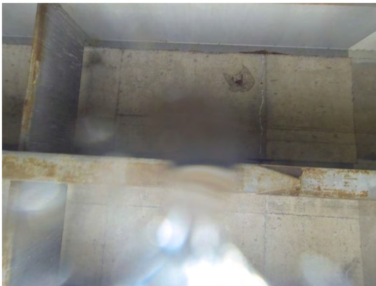
Figure 53: Example photo taken with the top-mounted, upwards facing GoPro while the Splash UAV performed a powered float underneath the test bridge, providing imagery of a spall despite the lens cover being wet.
