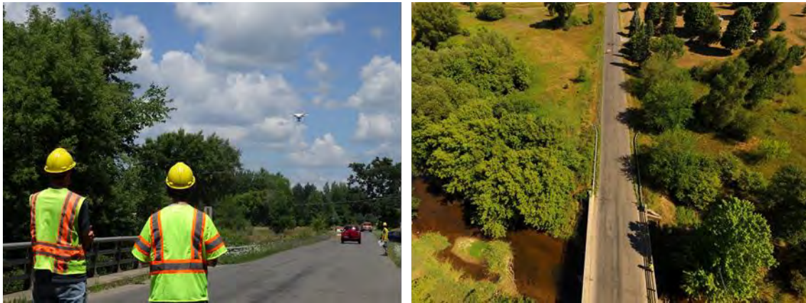
Figure 1: Collecting imagery data of the South Warren Road over Maple River bridge site (left) and example UAV image of the site (right) used to help create an overview image.
