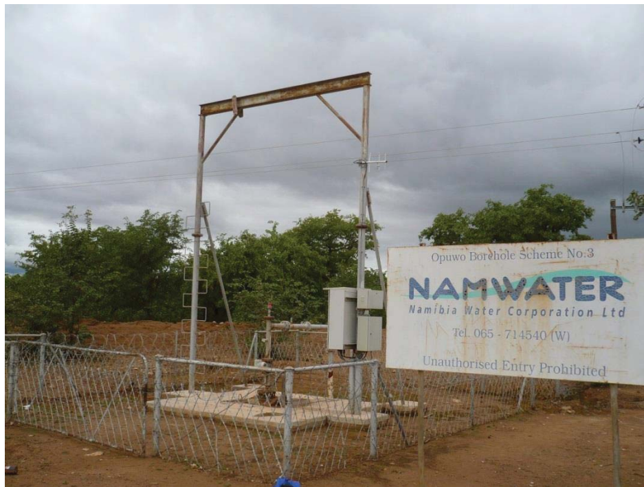
WW29045, characteristic of boreholes construction in the NW wellfield
