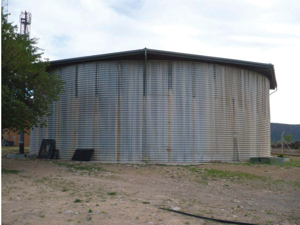
Storage Tank for Opuwo water distribution system
