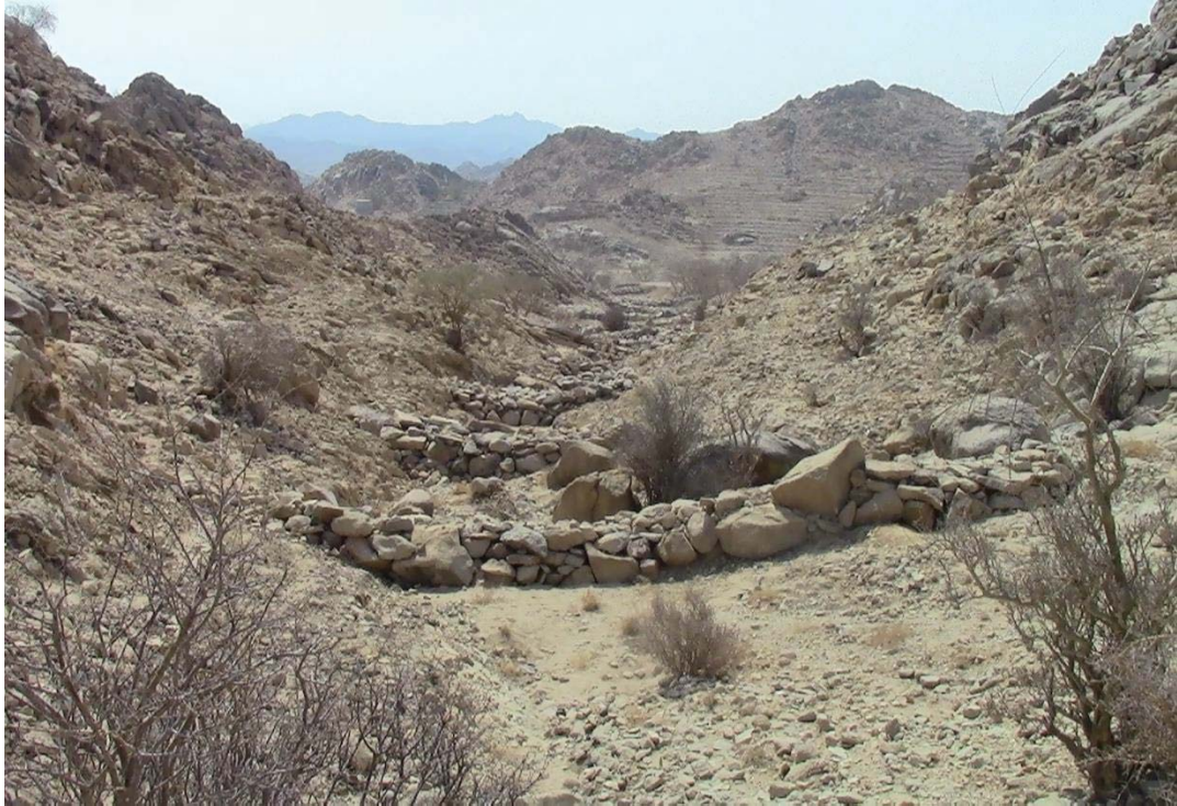
Figure 27: Check dam (photo adapted from http://www.permies.com/t/18489/desert/ready-plant-desert-south-Makkah )
