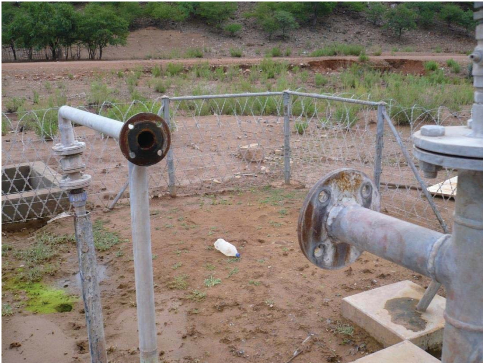
WW29047 under maintenance (2/24/2014)
