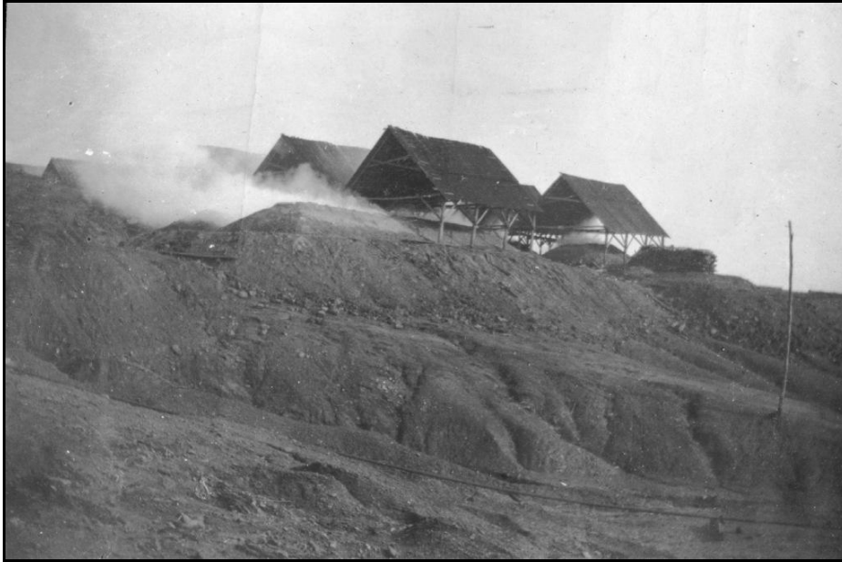
Figure 4.9 Open heap roasting in the Ducktown District ca. 1900. Large heaps of sulfur-rich copper ores, partially covered, were ignited on a bed of wood and allowed to burn for several weeks as most of the combustible sulfur burns off. (With permission of the Edward Oscar Boak collection, Ducktown Basin Museum.)
