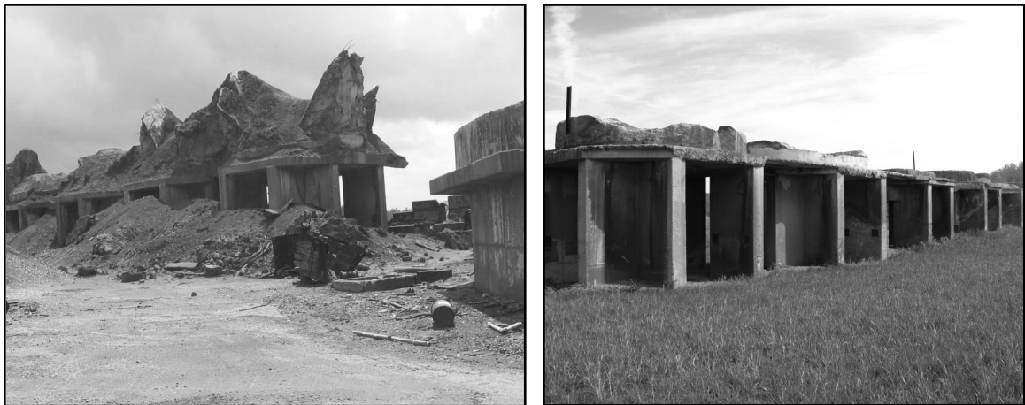
Figure 5.6 Fine Ore Bins at the London Mill site before restoration (ca. 2000) and after in 2008. (Sources left: EPA “Copper Basin Mining District Case Study: Use of Cooperative Agreements toward a Common Goal,” (2005), 1 and right: Author)
