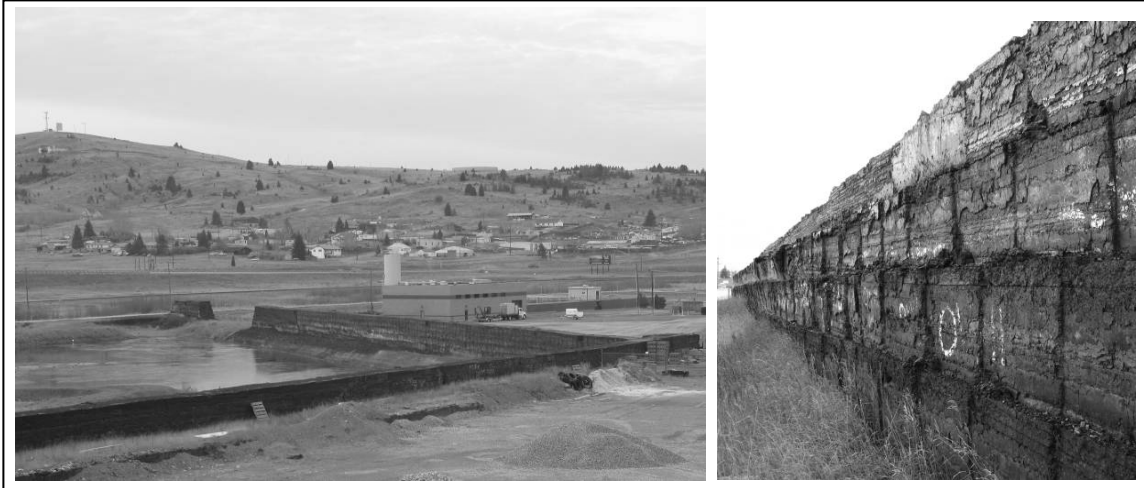
Figure 6.6 Slag walls of the Butte Reduction Works, 2008, showing former enclosed tailings ponds and close up of unique slag wall construction technique. (Source: Author)
