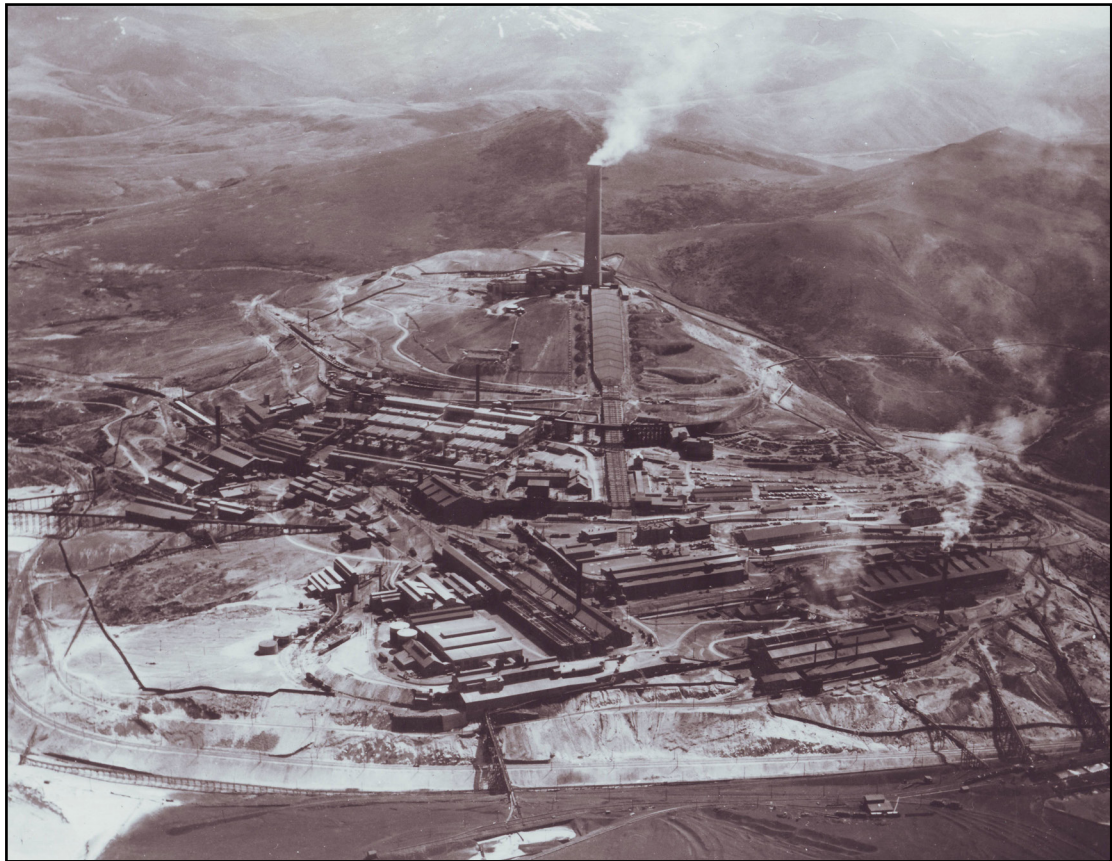
Figure 4.16 Anaconda Washoe Smelter ca. 1950s with separate concentrating, roasting, reverberatory furnace, zinc, leaching, and blast furnace buildings on the hill side and arsenic recovery, dust collection, and smoke stack on the hill top linked by a flue. (With permission of Marcus Daly Historical Society)
