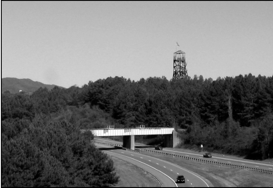
Figure 5.9 Central Shaft 2008 towering above State Highway 68 between Ducktown and Copperhill, Tennessee. (Source: author)
