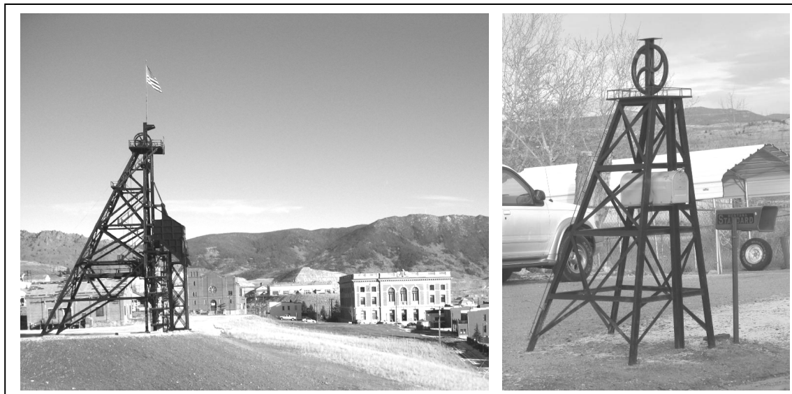
Figure 6.2 Gallows Frames of the Original Mine in Butte (left) and model frame used as a mailbox stand in the Flats (right). (Source: Author)
