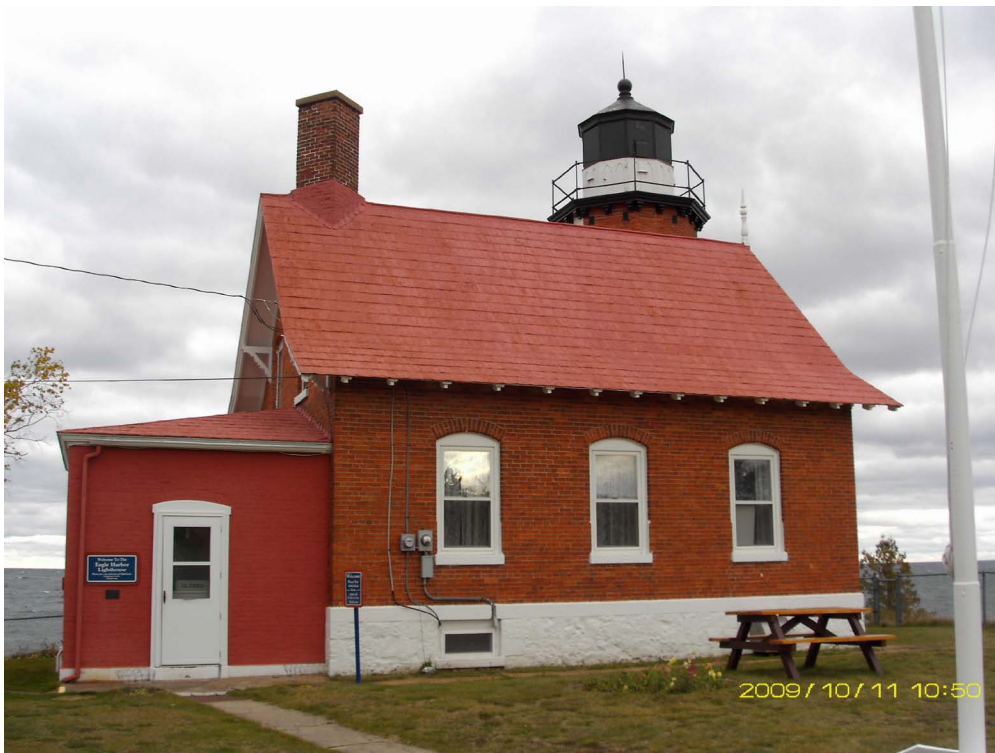
Figure III.4: Photograph of the current Eagle Harbor lighthouse structure. (Lisa Gillis, October 11, 2009.)
