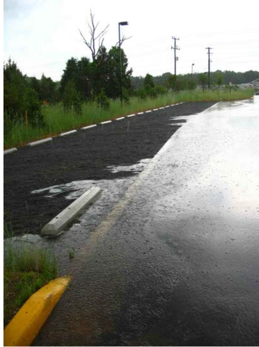
Figure 34. Runoff across watershed monitored at measurement point DP3, illustrating the high infiltration rate of Gravelpave2 porous pavement (left in photo) receiving runoff from the impervious asphalt (right in photo). The flow bypassing the DP3 monitoring point between the parking abutment and the orange curb is also evident, (Copyright 2006, Wetland Studies and Solutions, Inc.).
