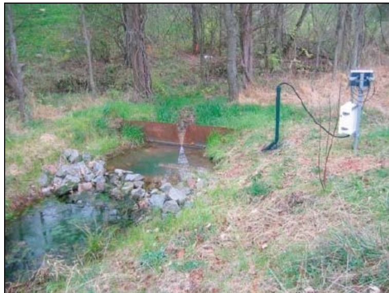
Figure 15. Thirty-degree V-notch weir and Model 8000 depth sensor installation with power and communication hookup. Photo taken in November 2006, (Copyright 2006, Wetland Studies and Solutions, Inc.).
