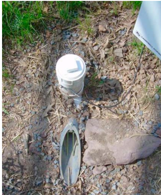
Figure 12. Grate replaced at DP3 (and DP4) in Spring 2007, Rat Guards™ by AgriDrain Cooperation models RG06 and RG04, respectively. Photo taken April 2007, (Copyright 2007, Wetland Studies and Solutions, Inc.).
