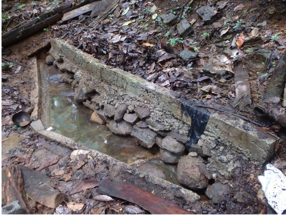
Figure 5: Picture of the spring box and seepage spring for this study (Photo taken by author)
