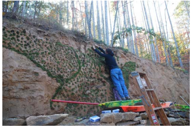
Figure 60. Coworker inserting mosses in depressions made for the moss. Photo courtesy of Annie Martin.
