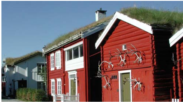
Figure 82. Buildings in Norway with natural green roofs. Photo by Michael Lüth, with permission.
