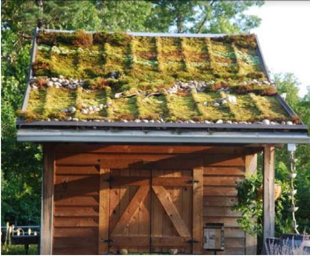
Figure 98. Moss roofing completed. Photo by Annie Martin, with permission.
