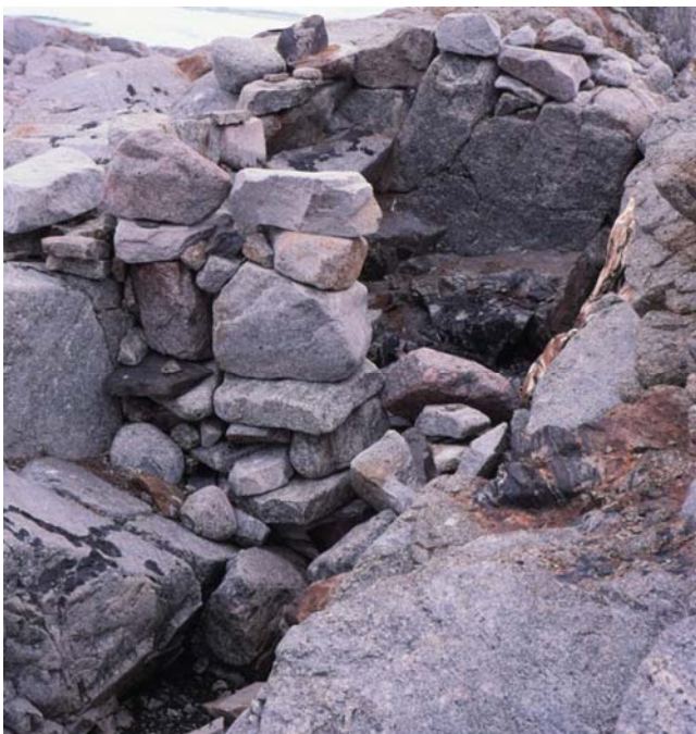
Figure 5. Remains of Granite House, with moss chinking, at Cape Geology, Antarctica. Photo by Rod Seppelt, with permission.
