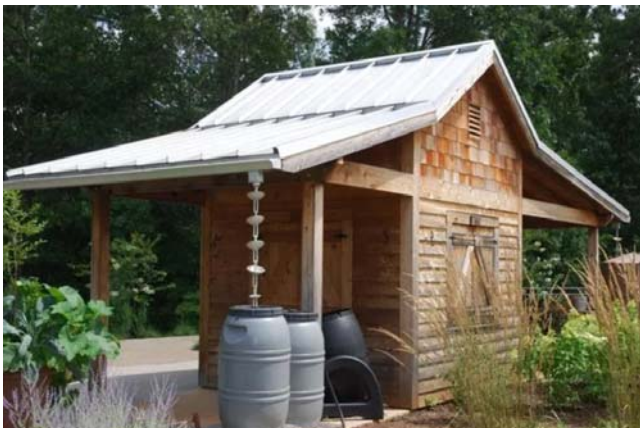
Figure 94. Experimental moss roof before application of mosses, North Carolina Arboretum in Asheville, NC, USA. Note the rain barrels already collecting rainwater for watering the mosses when they are planted. This building and its rainwater collection system is a demonstration experiment for the botanical garden. Photo by Annie Martin, with permission.
