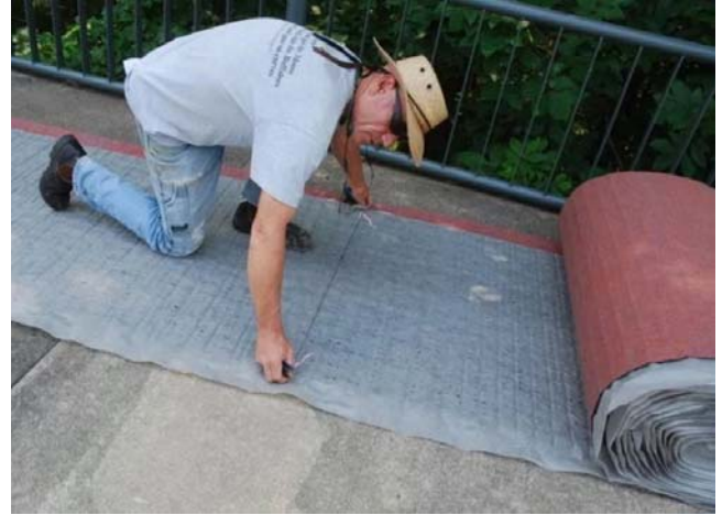
Figure 95. Moss roofing, preparing the substrate. Photo by Annie Martin, with permission.
