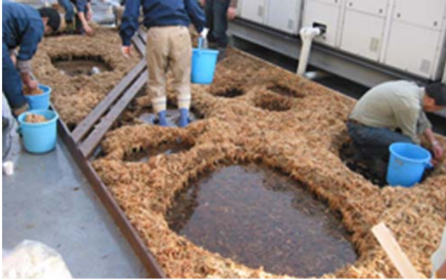
Figure 92. Maintaining Sphagnum bog for roof. Photo courtesy of Hironori Deguchi.
