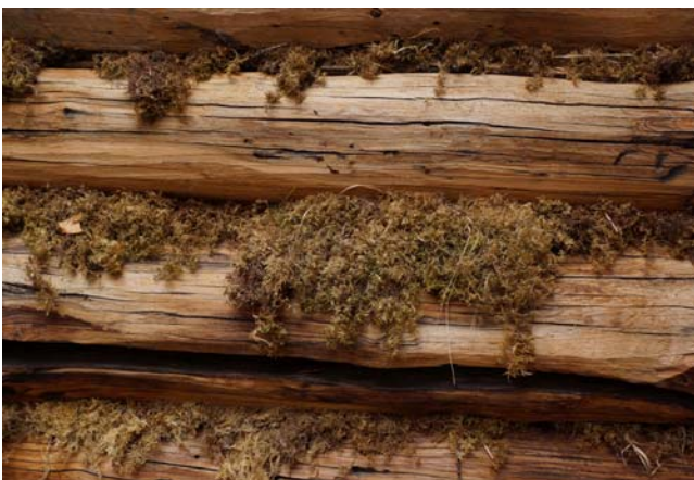
Figure 22. A log house that has caulking (chinking) with Hylocomium splendens in China. Photo courtesy of Li Zhang.
