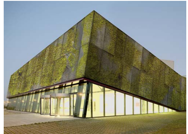
Figure 36. Centro Cultural Aeronáutico, Barcelona, showing biological concrete. Photo from Escofet 1886, S.A., courtesy of Sandra Manso Blanco.
