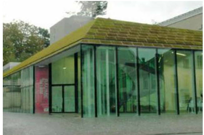
Figure 70. This modern building has a green moss roof. Photo courtesy of Michel Chiaffredo.
