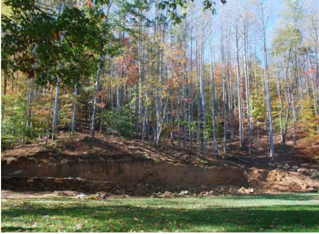
Figure 56. This recently cut clay bank is begging for erosion protection. The stone wall at the bottom will only catch the clay after it has been washed down. Photo from MountainMoss, courtesy of Annie Martin.
