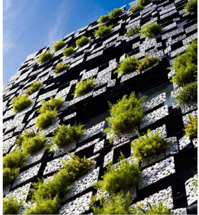
Figure 31. Closer view of living wall, dezeen Green Cast by Kengo Kuma. Photo courtesy of Sandra Manso Blanco.
