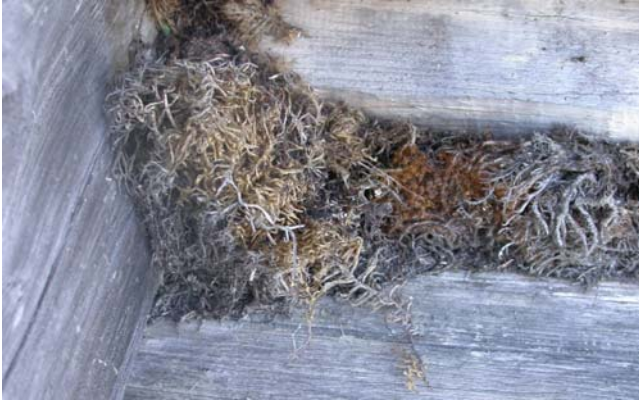
Figure 9. Moss chinking with a variety of species in a fishery hut on the dock near the Rock Harbor Light House, Isle Royale National Park, Michigan, USA. Photo courtesy of Diane Lucas.
