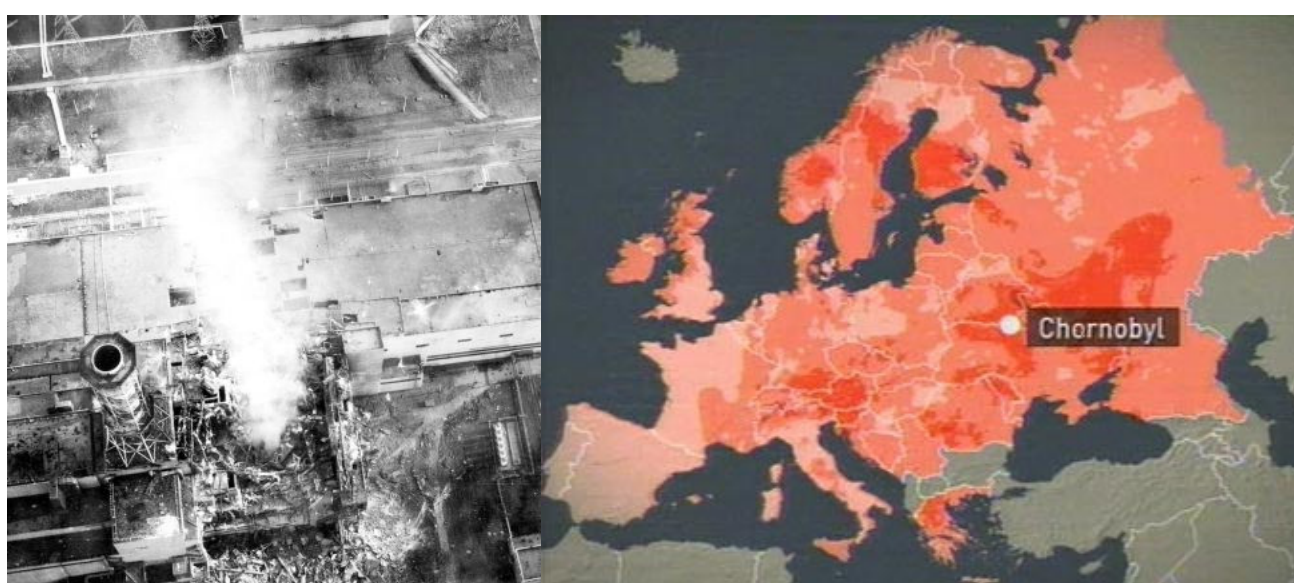
Figure 1. (a) Chernobyl aerial view into the core, smoke from the graphite fire and core melt down. The photo was taken from a helicopter on May 3, 1986, of the destroyed Unit 4. (b) Radiation fallout from Chernobyl [40].
