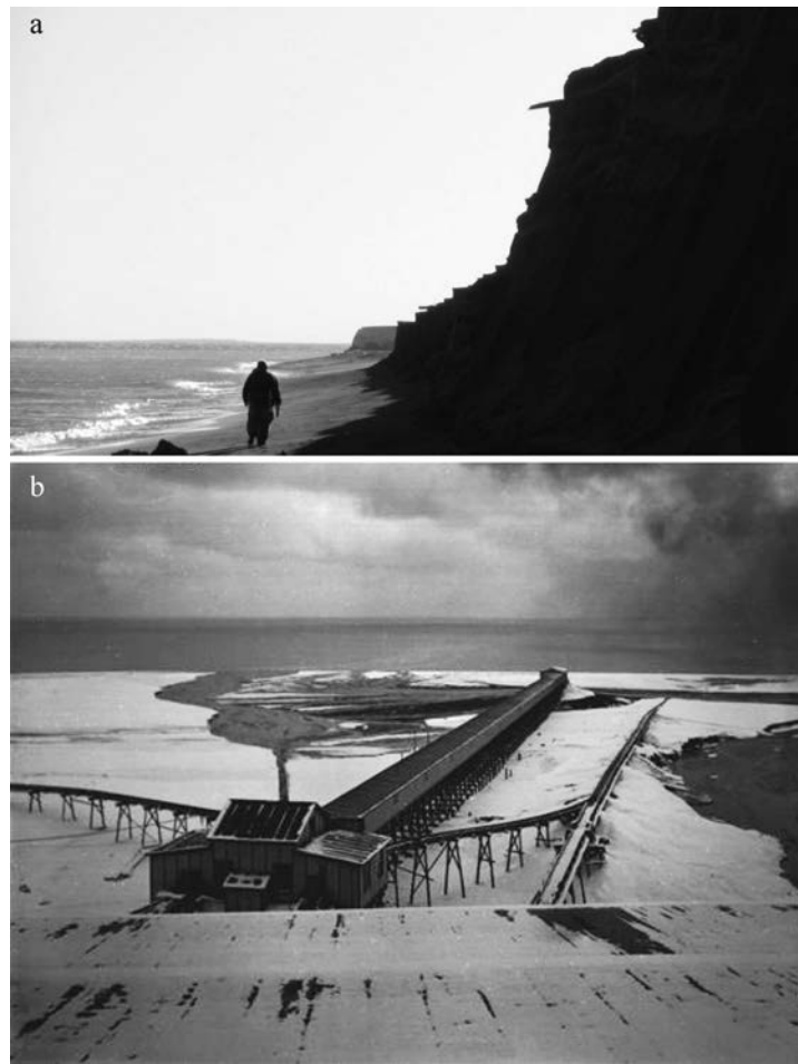
Fig. 7. (a) Wave erosion of the Gay tailings pile. The near-vertical 7-m bluffs contain well-preserved remnants of wooden troughs that sluiced stamp sands across the pile. (b) Primary and secondary sluiceways (Wolverine Mill, winter 1922) carry stamp sands over the Gay pile. Lake Superior is on the horizon. Notice melted regions with fresh discharges. Photo courtesy of Michigan Tech Archive.
